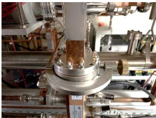
Fig. 5. New installed 7 th RF water loading
